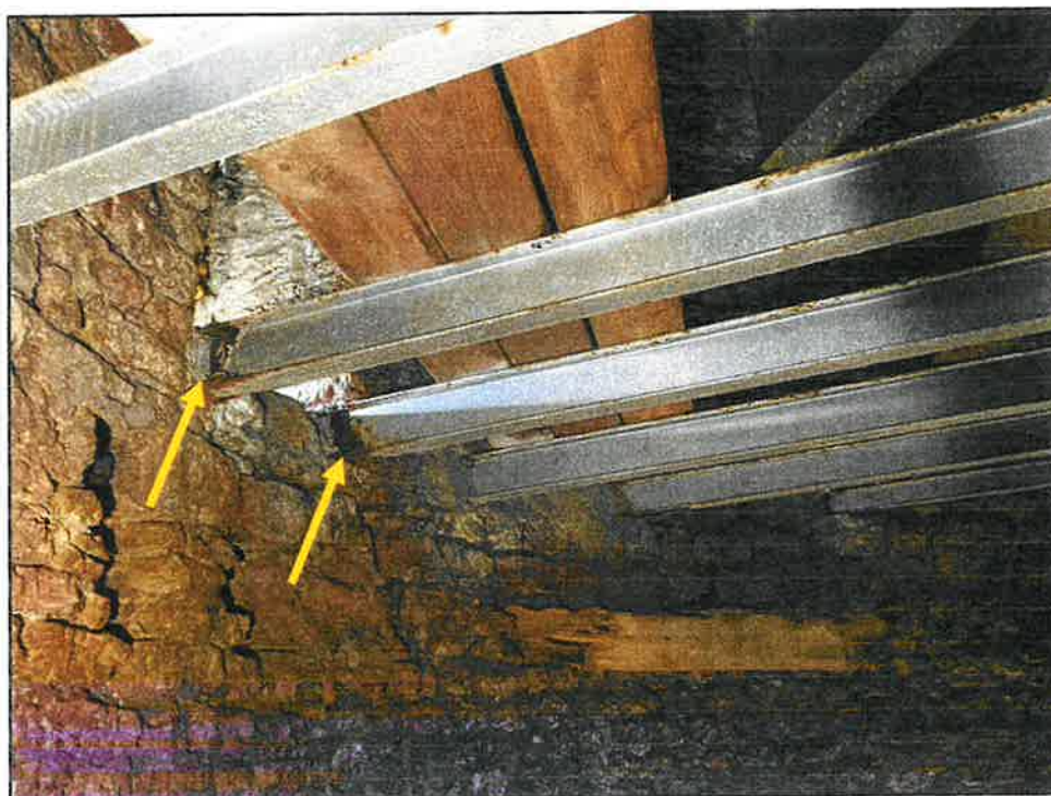
Photo 34: Signs of floor beam corrosion at walls
