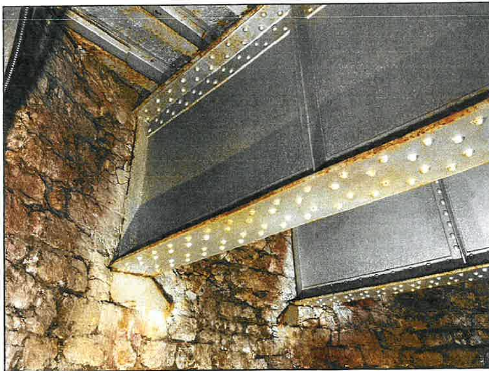
Photo 3: Steel plate girder supports
