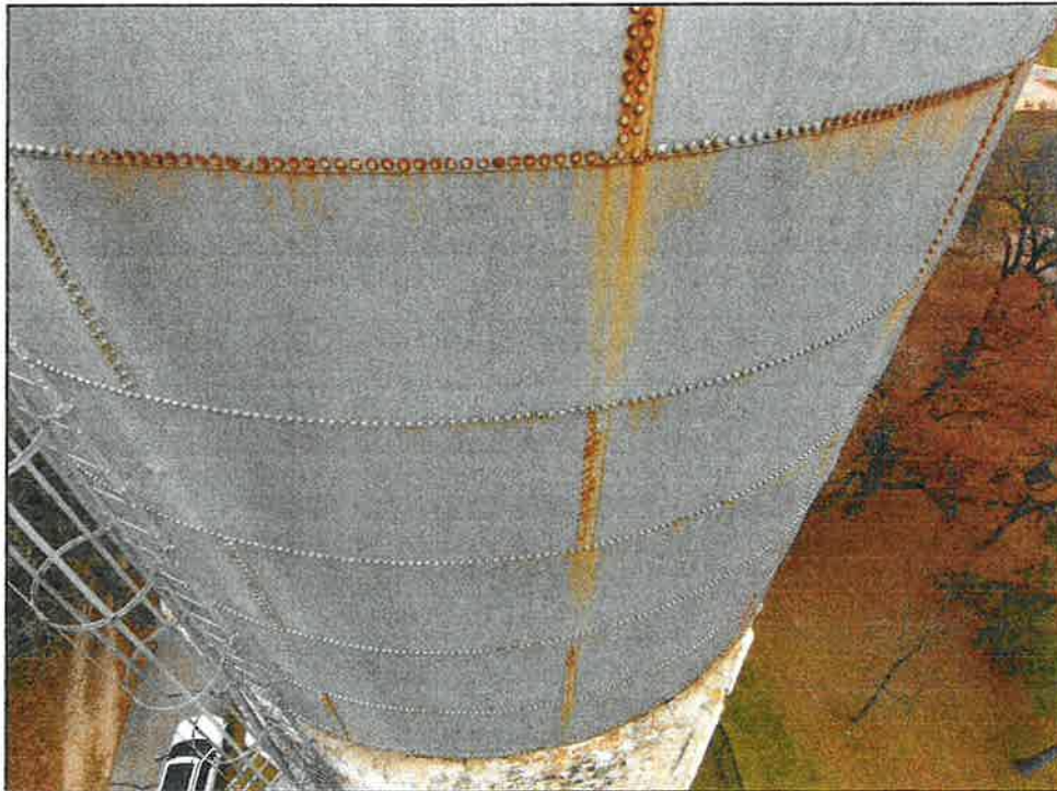
Photo 36: Rust staining on exterior of tank
