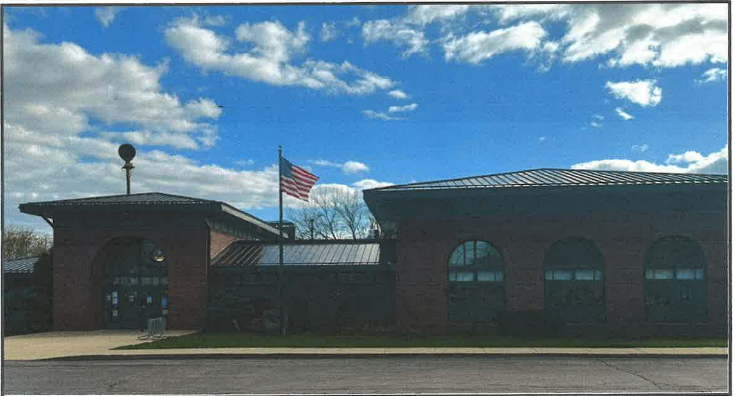
Shingle removal and replacement with a standing seam roof with matching snowguards. The flat roof was installed for 25 year NDL warranty - fully adhered EPDM. Project size: 15,000sf
