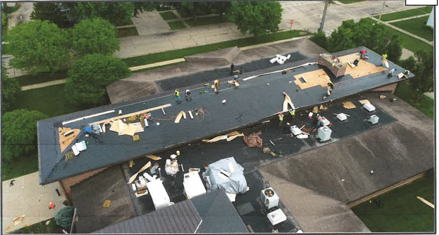
Shingle removal and replacement with a standing seam roof with matching snowguards. The flat roof was installed for 25 year NDL warranty - fully adhered EPDM. Project size: 15,000sf
