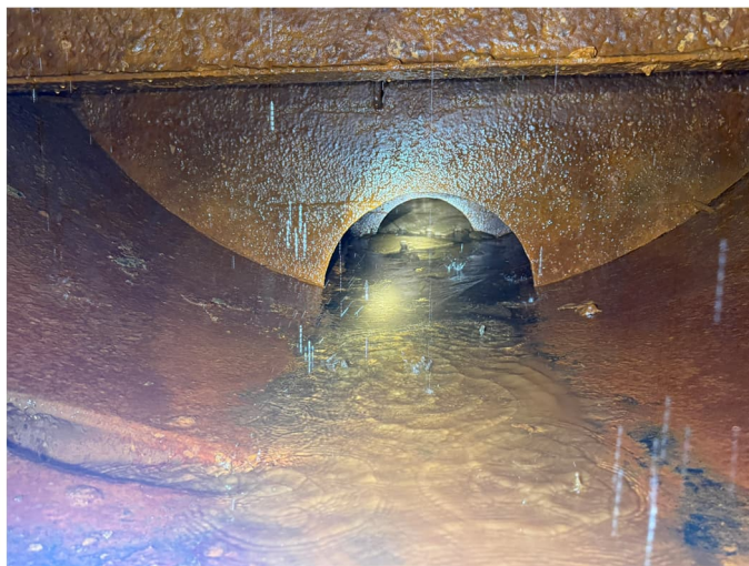
Figure 1 Filter Underdrain
