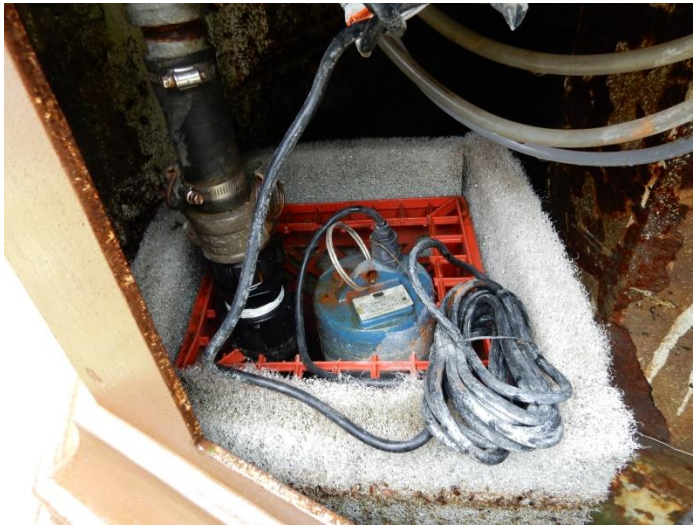
Image 12: Detail of Submersible pump
