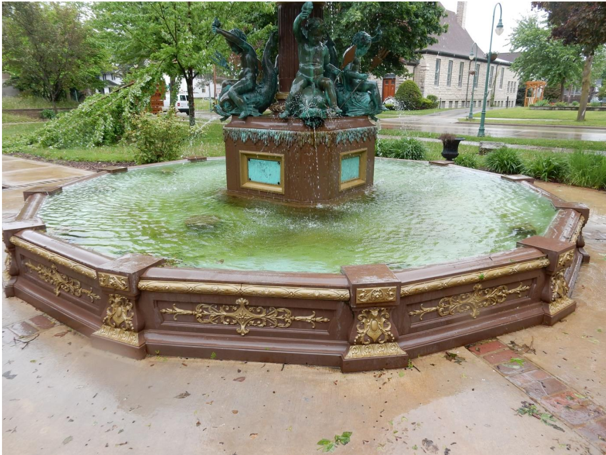
Image 02: Detail of Fountain Base
