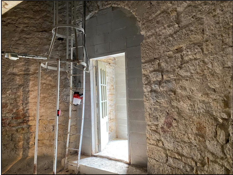
Photo 10: Modified entry door/wall
