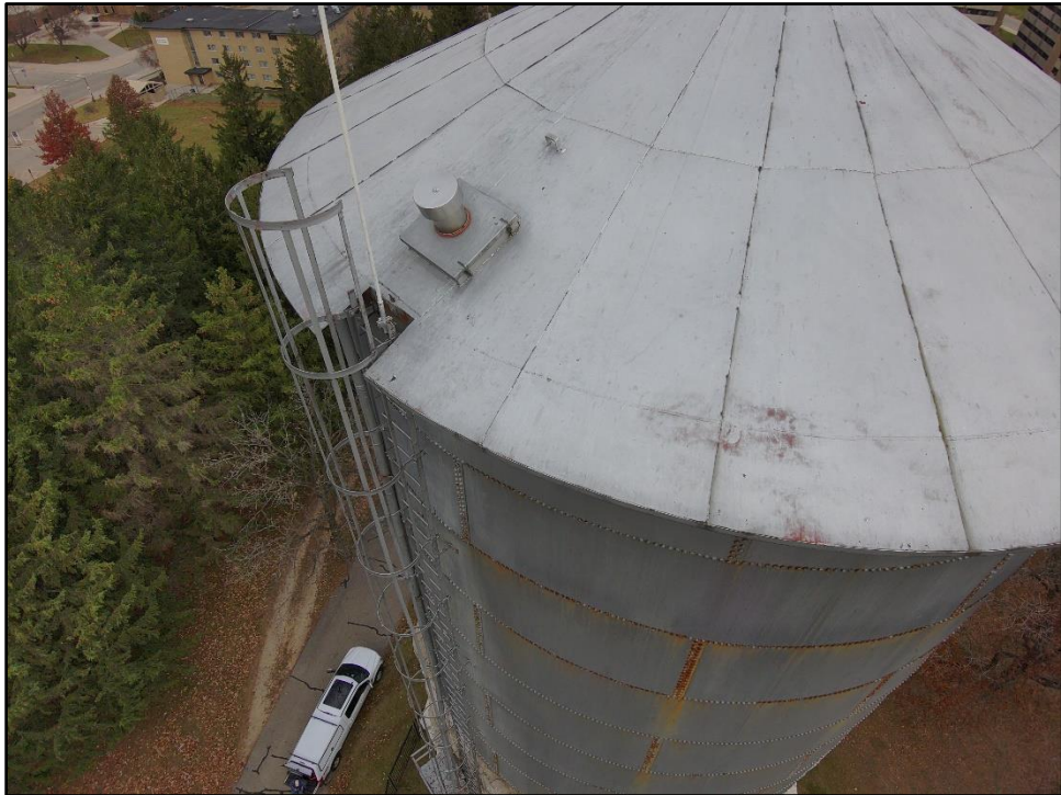
Photo 9: Exterior ladder to tank
