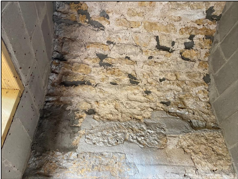
Photo 25: Different mortar at entry arch
