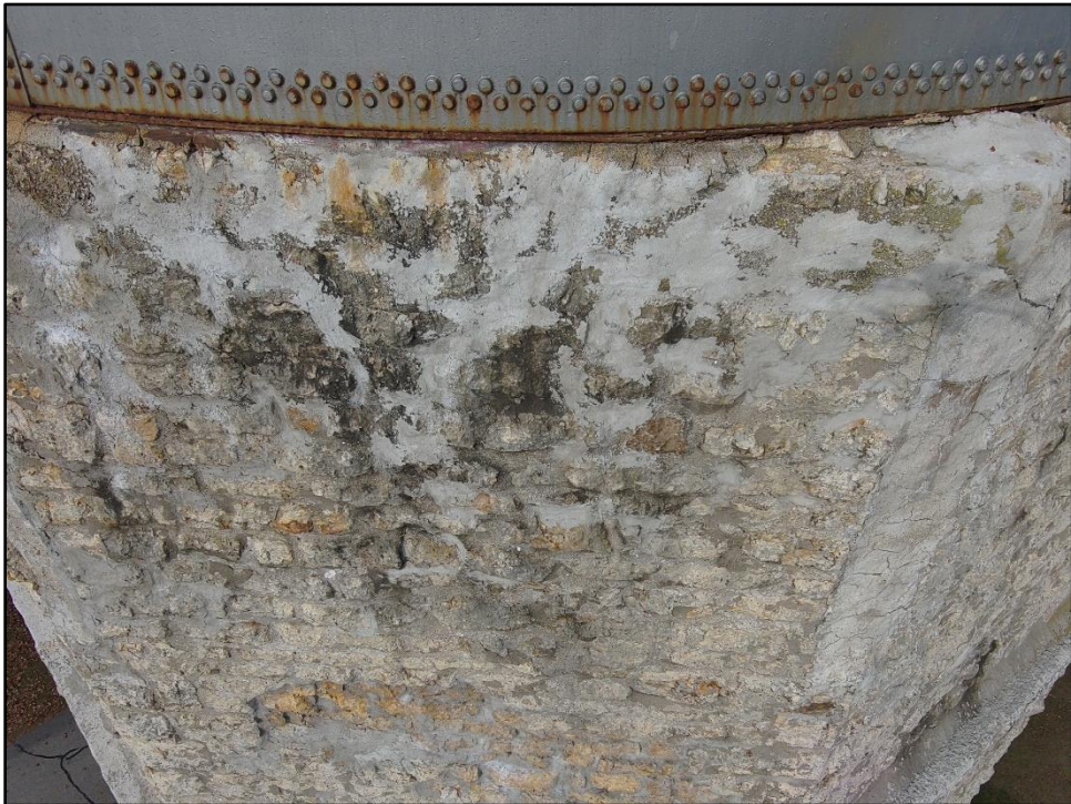
Photo 27: Repointing mortar at top of tower
