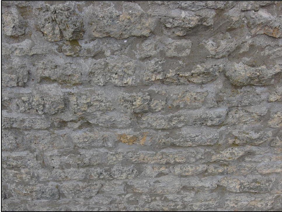
Photo 26: Repointed joints at mid-height of tower
