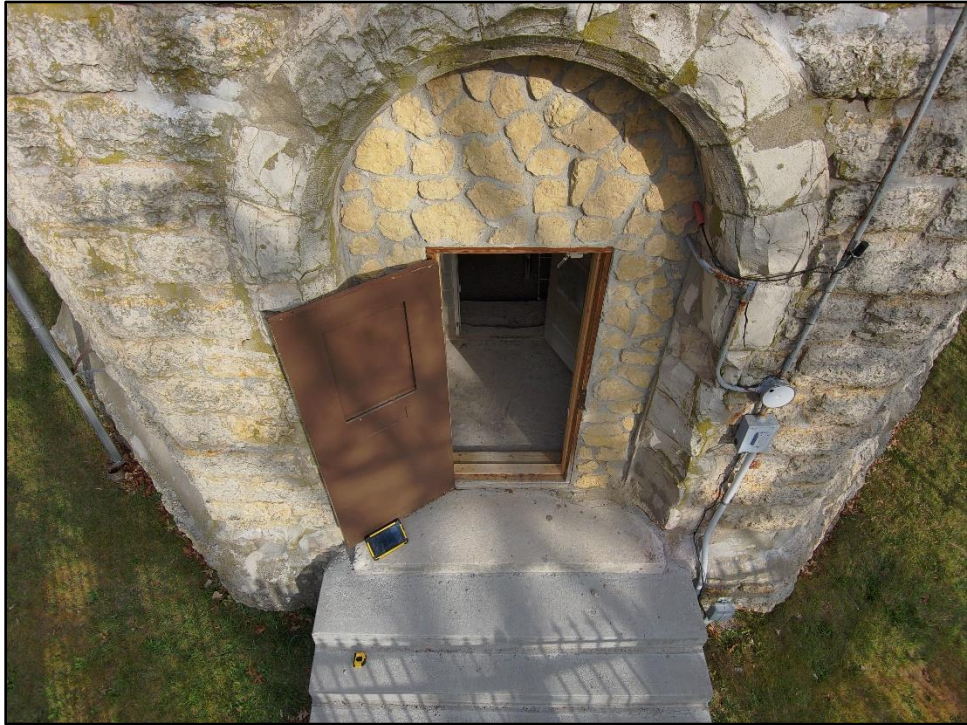
Photo 11: Modified entry door/wall
