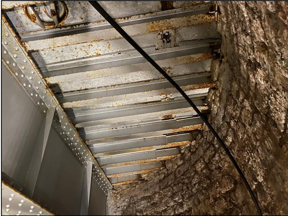
Photo 2: Steel beams below tank
