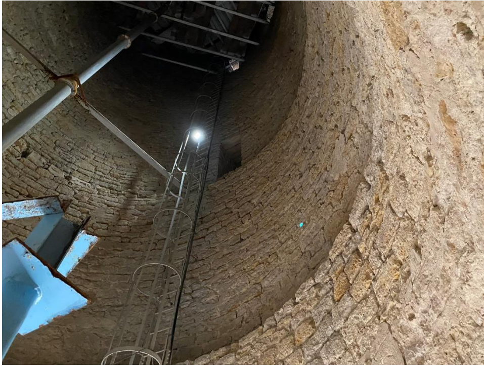
Photo 6: Ladder inside masonry tower
