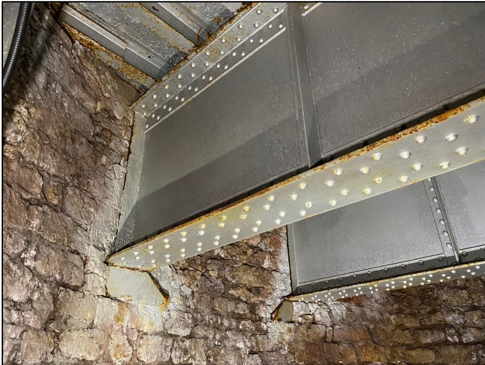
Photo 3: Steel plate girder supports
