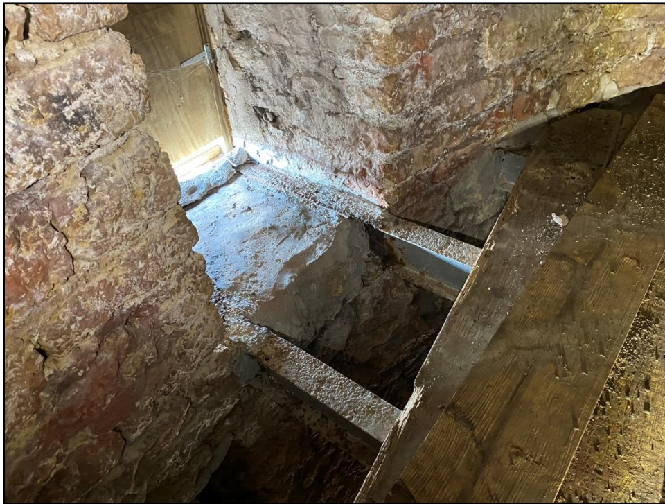
Photo 7: Doorway to exterior platform and ladder
