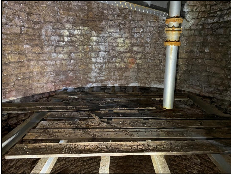
Photo 4: Floor below tank at top of masonry tower
