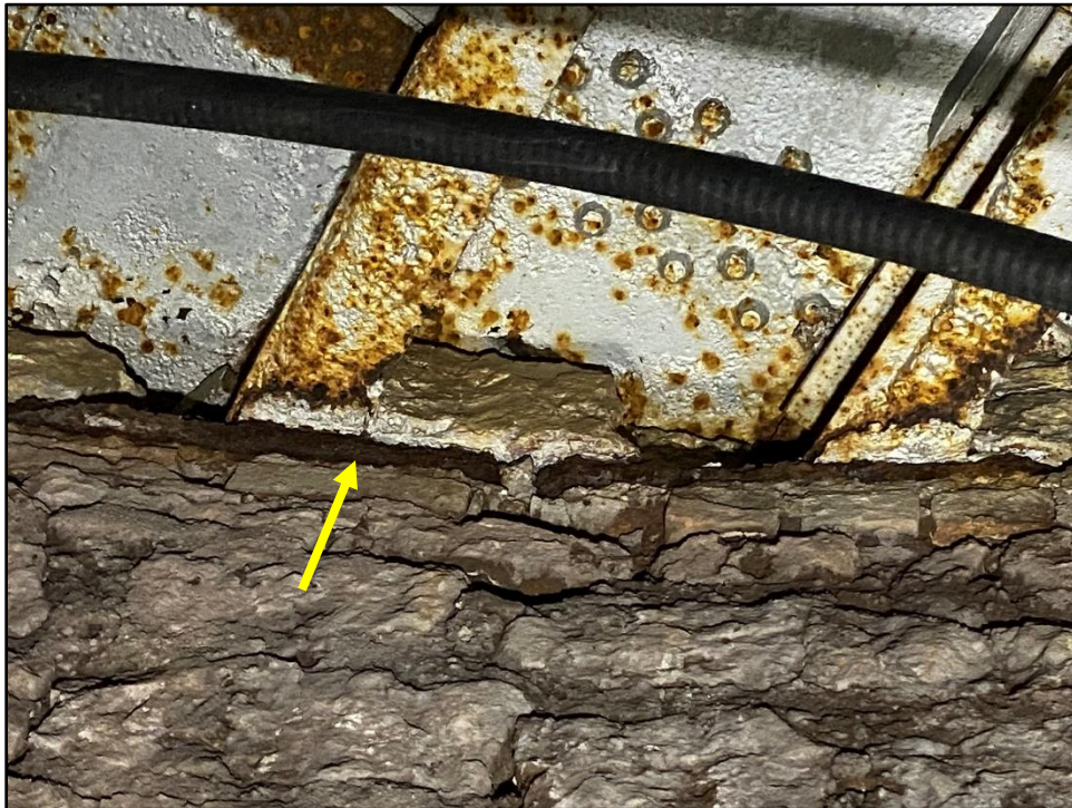
Photo 32: Close up of tank supports at wall
