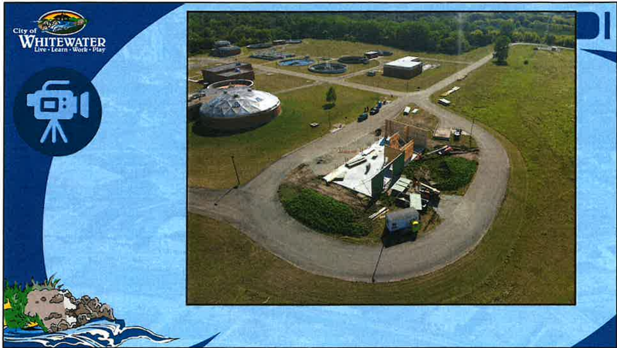
Picture above is an ariel shot of the progress on the new WPD Evidence Garage.
