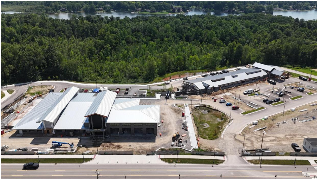
Aerial view of the new White Lake Township Civic Center Campus, under construction — August 21, 2026
