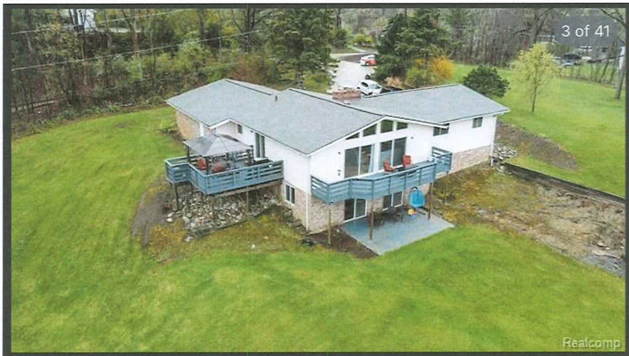
Figure 1 – Original rear elevation of the residence before renovations.
