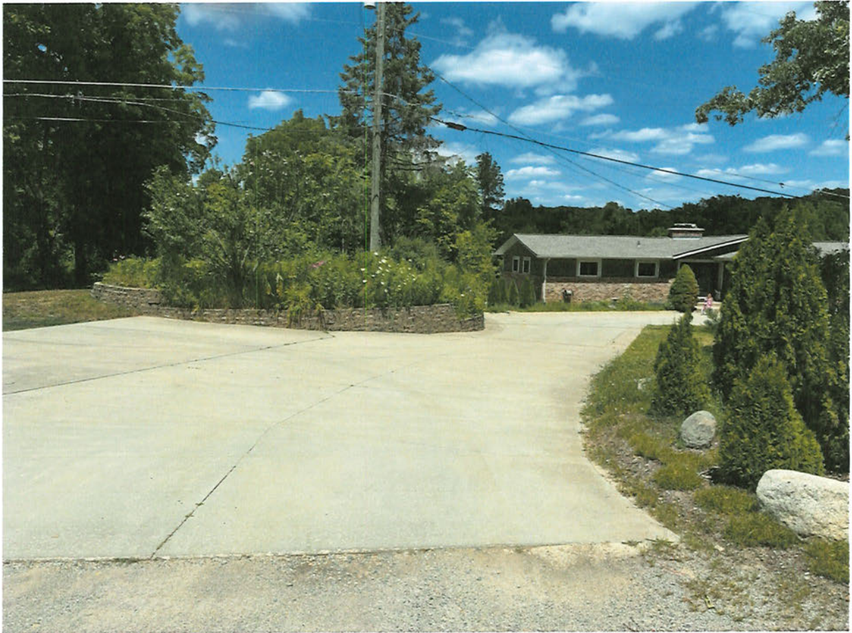
Figure E-2 – Concrete Driveway Entrance
