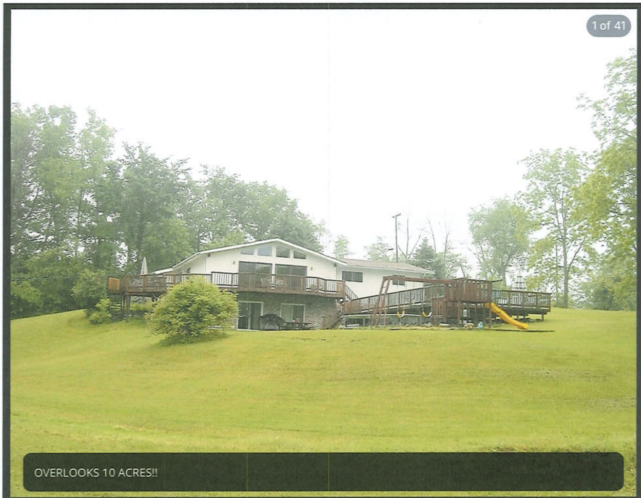
Figure 6 – Rear elevation prior to renovation.
