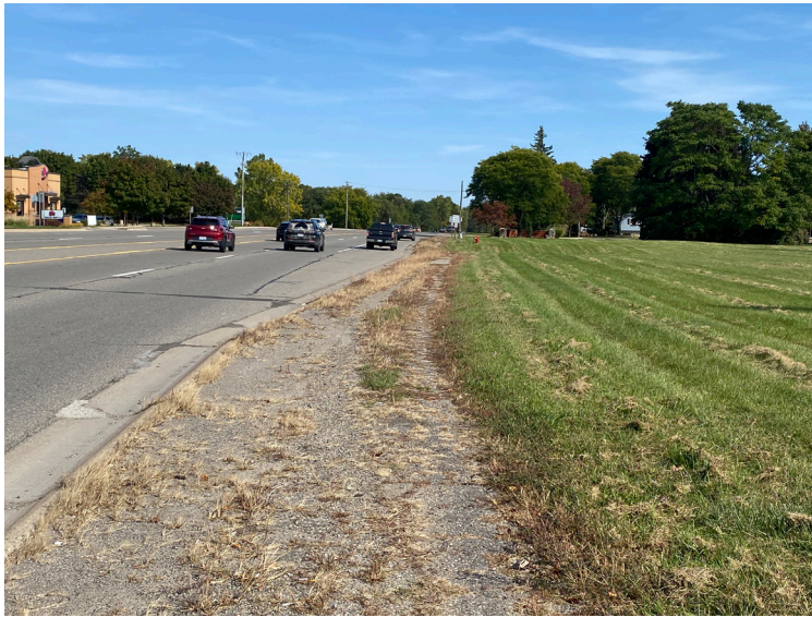
Aging and unkempt asphalt along edges of M-59
