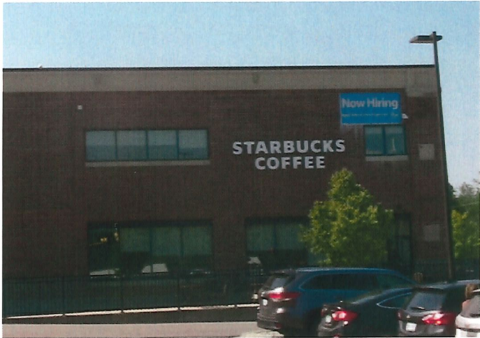
EXISTING SCOPE OF WORK: FRONT ELEVATION - REMOVE AND INSTALL NEW STARBUCKS DISK.
