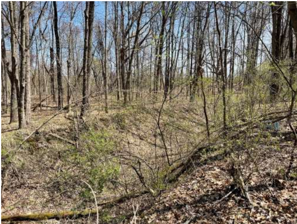
Photo 7. View of constructed upland ditch on the eastern edge of the AOI.
