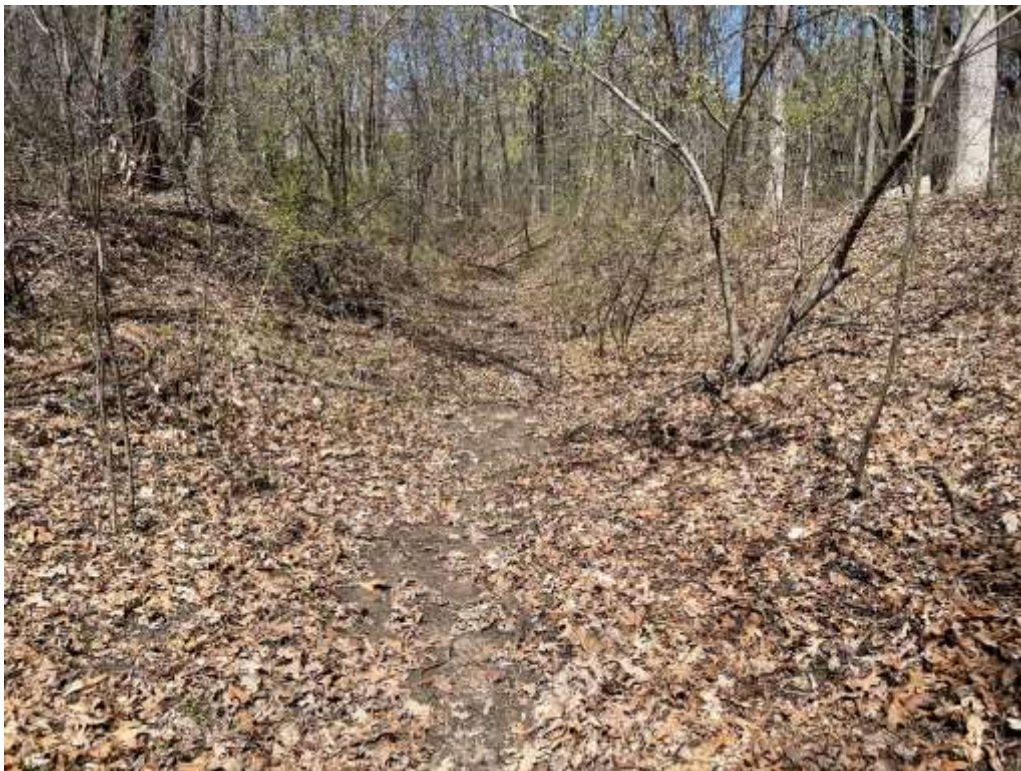
Photo 8. Additional view of upland constructed ditch on the eastern edge of the AOI.
