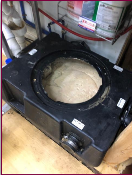
Standard In-Kitchen Grease Control Device
