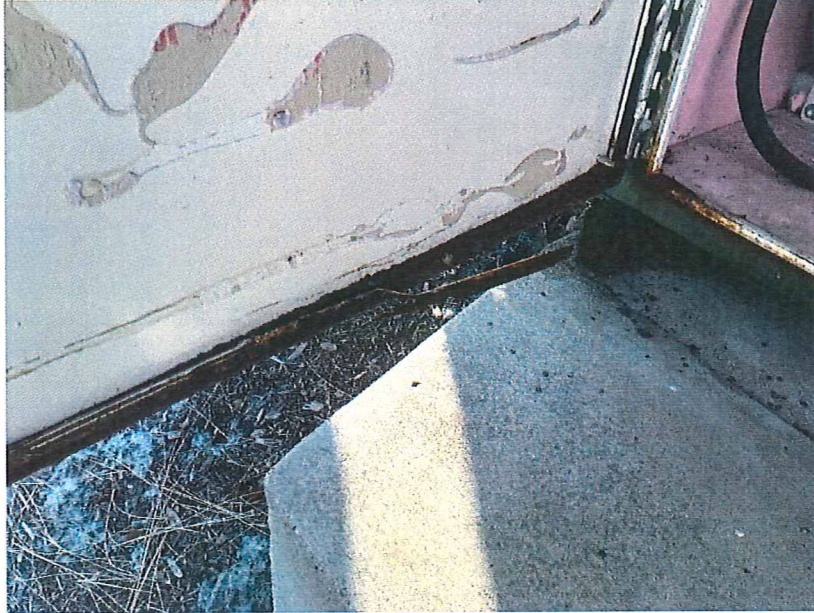
Figure 2 - Marketplace Lift Station Cabinet Corrosion
