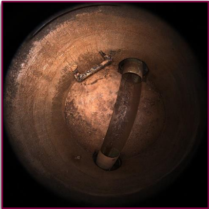
Wastewater Manhole Structure
