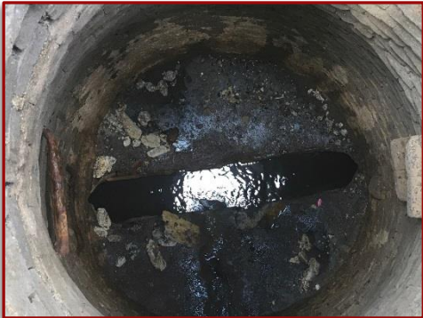
Wastewater Manhole Structure
