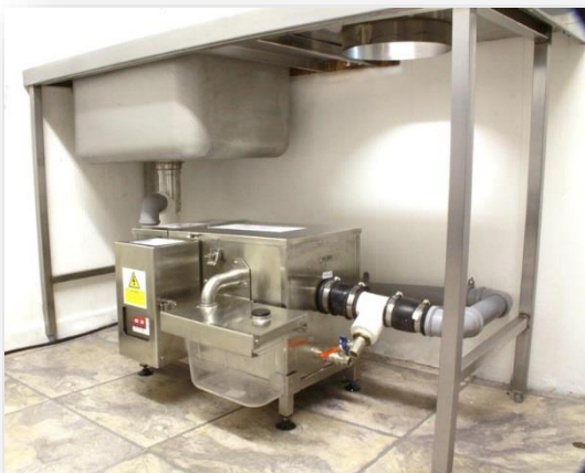
Grease Trap (Under the Sink) Example
