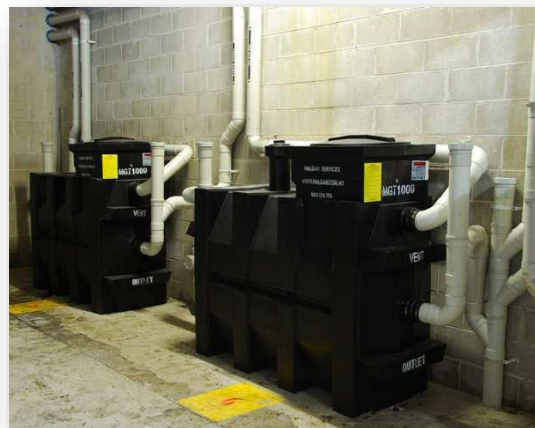
Grease Interceptor (In Basement) Example
