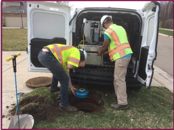
Figure 20 Manhole Scanning
