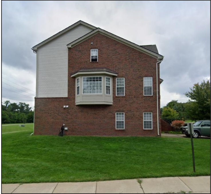
Existing Condominium Building
