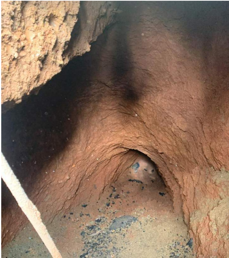
Photo 5: Brick Exposed at End of Tunnel
