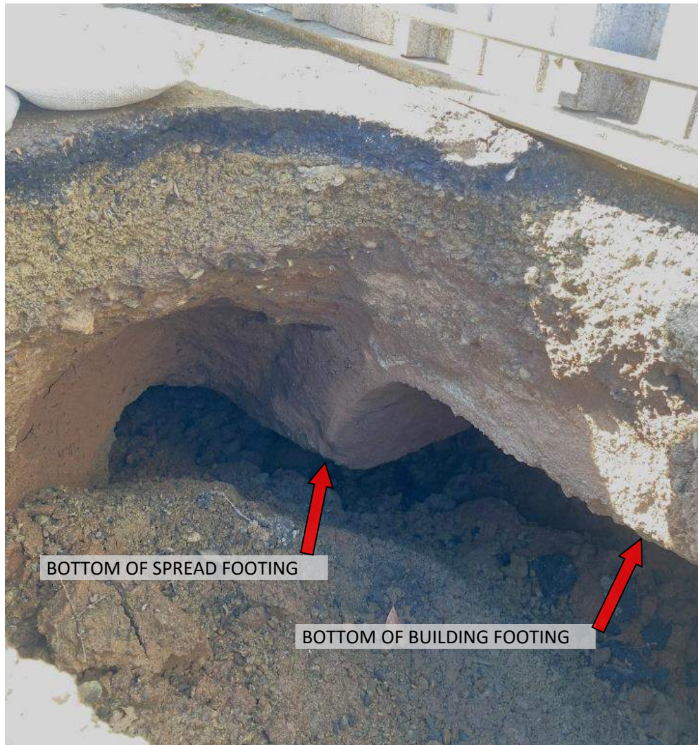
Photo 3: Exposed Foundation and Spread Footing, Tunnel to the Southeast of the Hole
