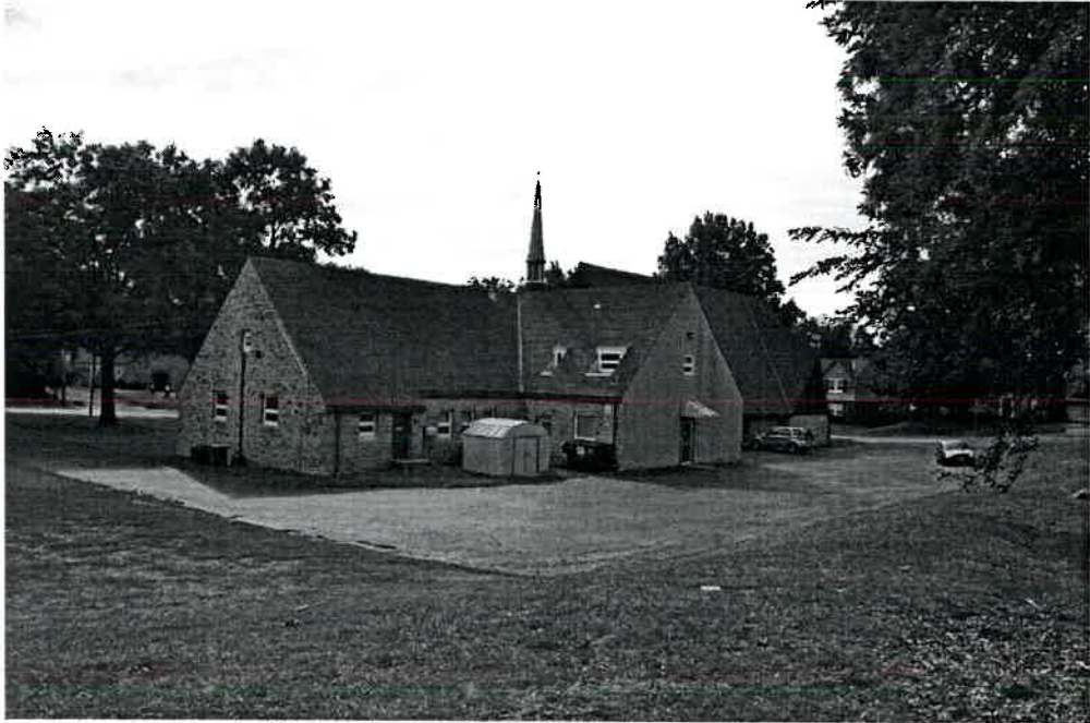
Looking southeast at the northwest elevation of the building
