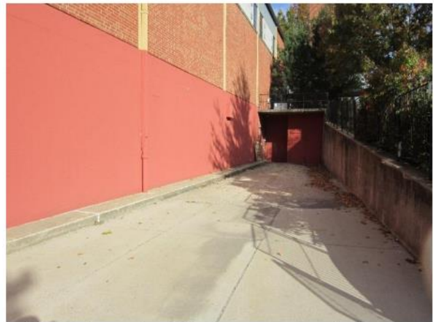
Additional exterior lighting recommended for security.
