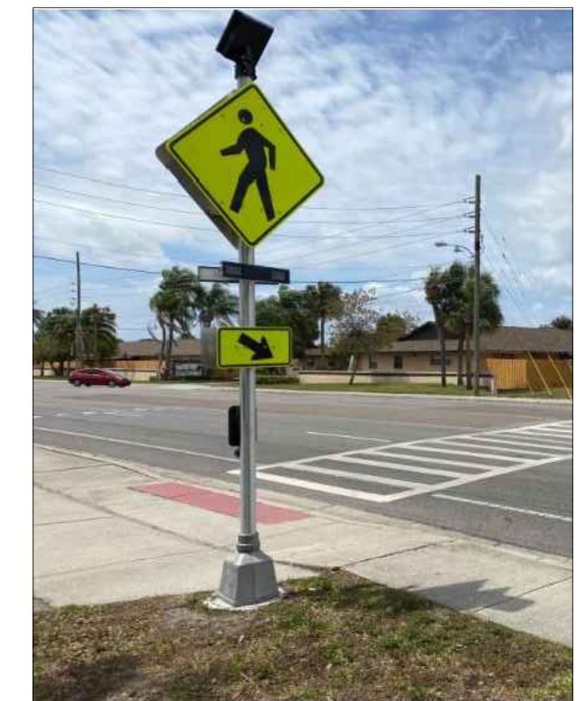
Rapid Repeating Flashing Beacon (RRFB)
