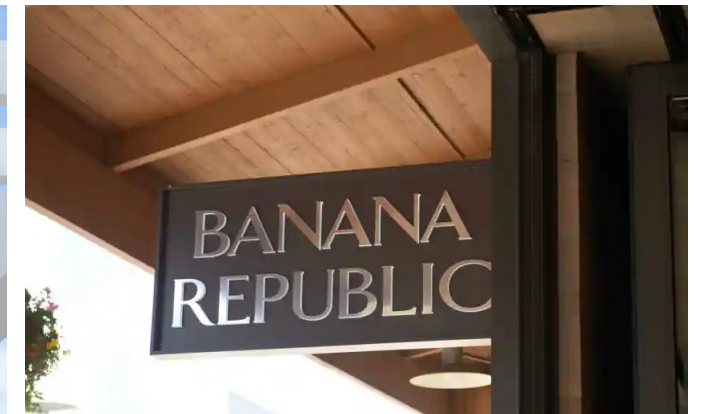
Pushed through sign panel
