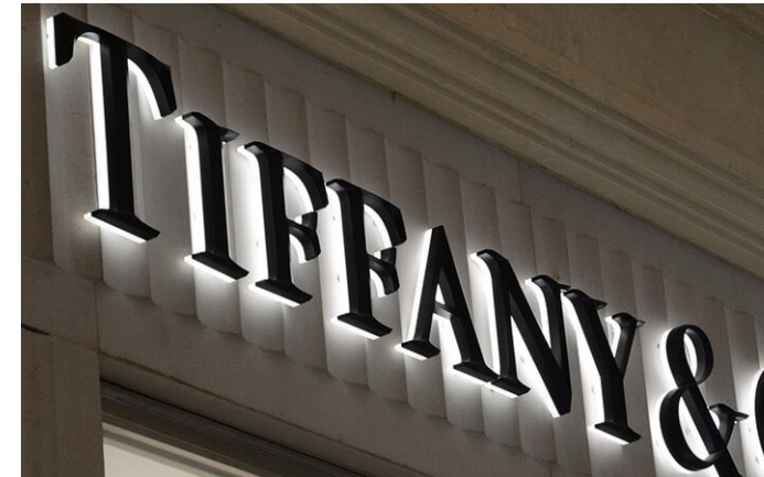
Flat cut out pin-mounted halo-lit letters
