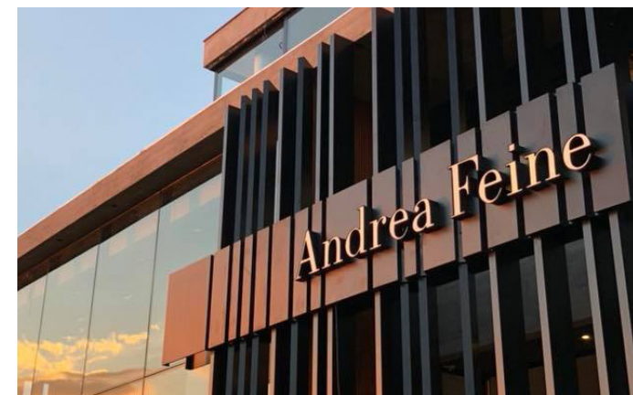
Fabricated letters integrated into architecture
