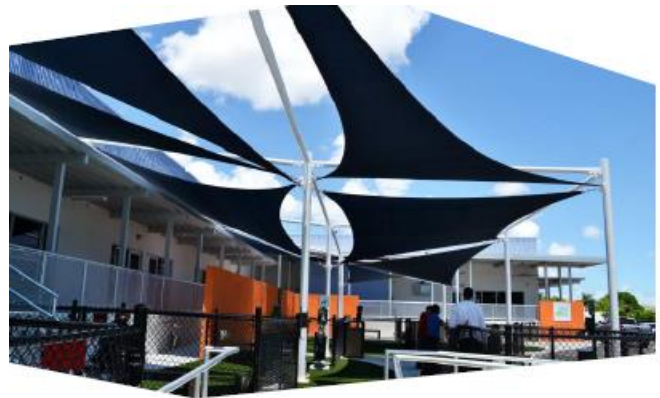
Pit Lane Shade Structure
