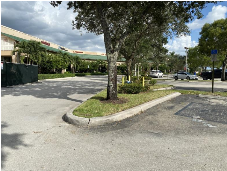
Example of 9" DBH Live Oak in narrow terminal island with insufficient curb radii. Radii will be fixed and trees saved in most cases.
