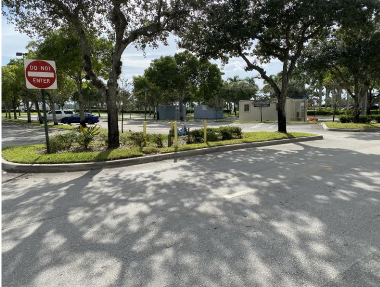
Example of 8-10" DBH Live Oaks in terminal island noting poor pruning activities. The majority will be saved.
