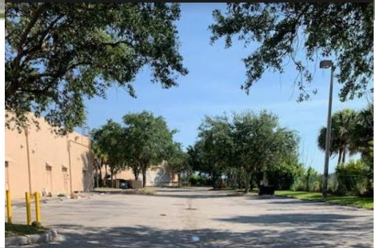
Plaza rear area provides space for tents and tables without conflicting with Fire Lne
