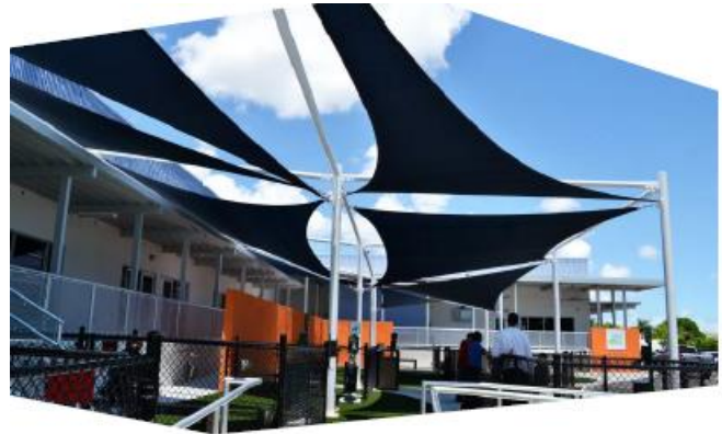
Pit Lane Shade Structure
