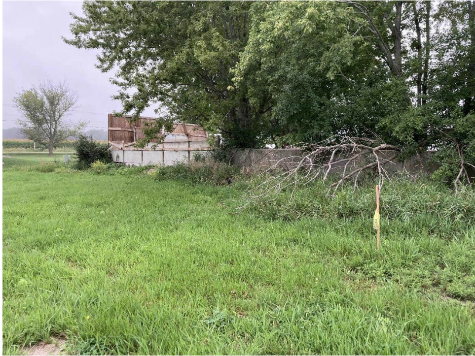
Looking NW at abandoned building
