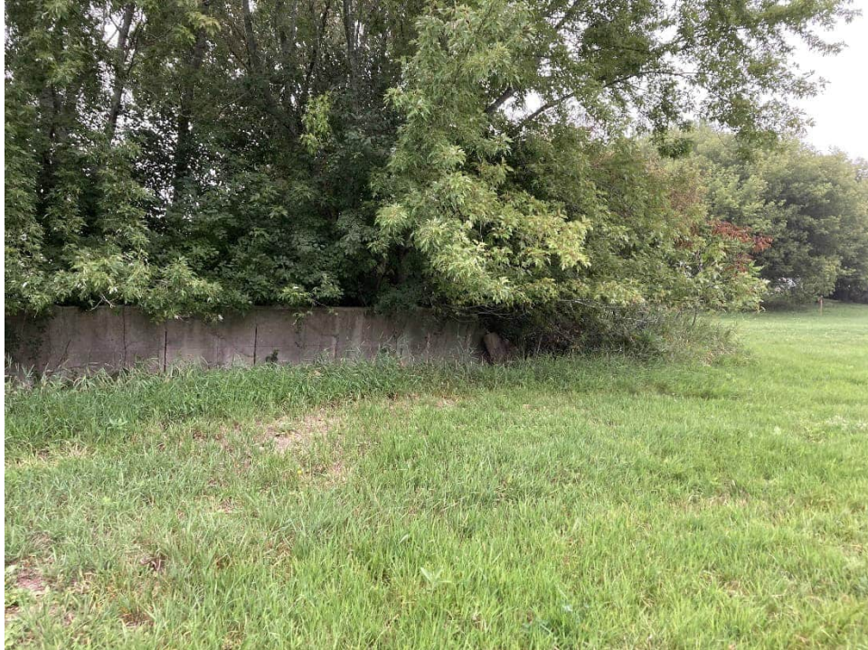
Looking NE at abandoned building
