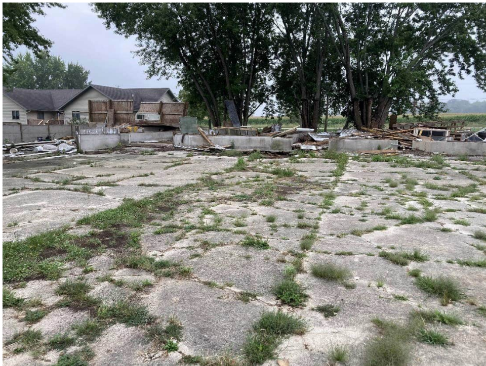
Looking W at abandoned building
