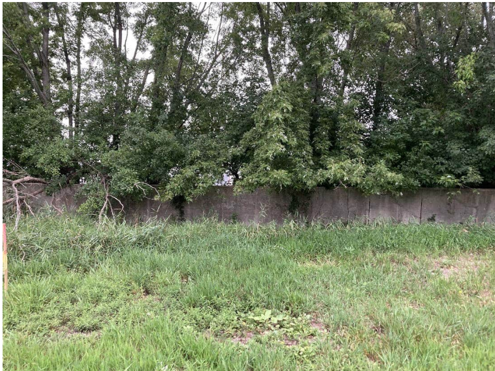
Looking N at abandoned building
