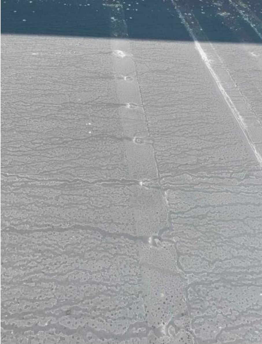
Rubber Roof No damage
