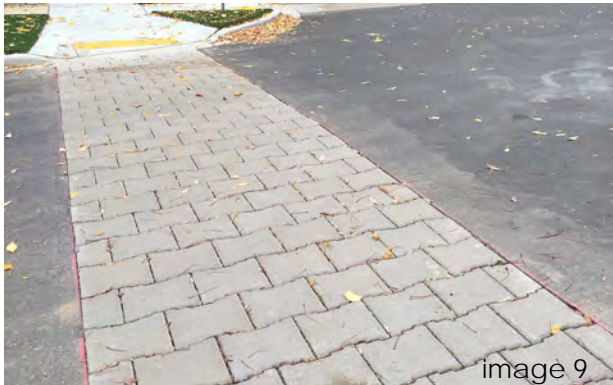
Above: Pervious pavers integrated into crosswalk (left) and parking spaces (right).
