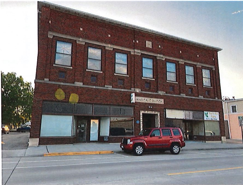
Building photo. The yellow dots are proposed locations for the exterior sign.
