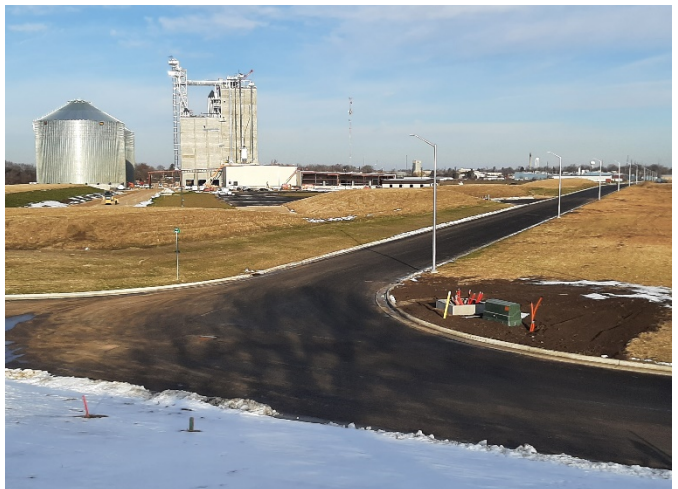
After Construction – At Shaler Dr. & Wilson Dr. intersection (Looking North)
