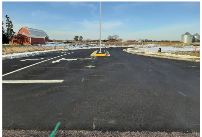
After Construction – At S.T.H. 26 and Shaler Dr. intersection (Looking West)
