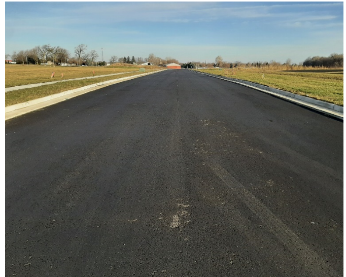
After Construction – At Shaler Dr. & Bayberry Ln. intersection (Looking North)
