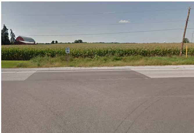
Before Construction – At S.T.H. 26 and Shaler Dr. intersection (Looking West)
