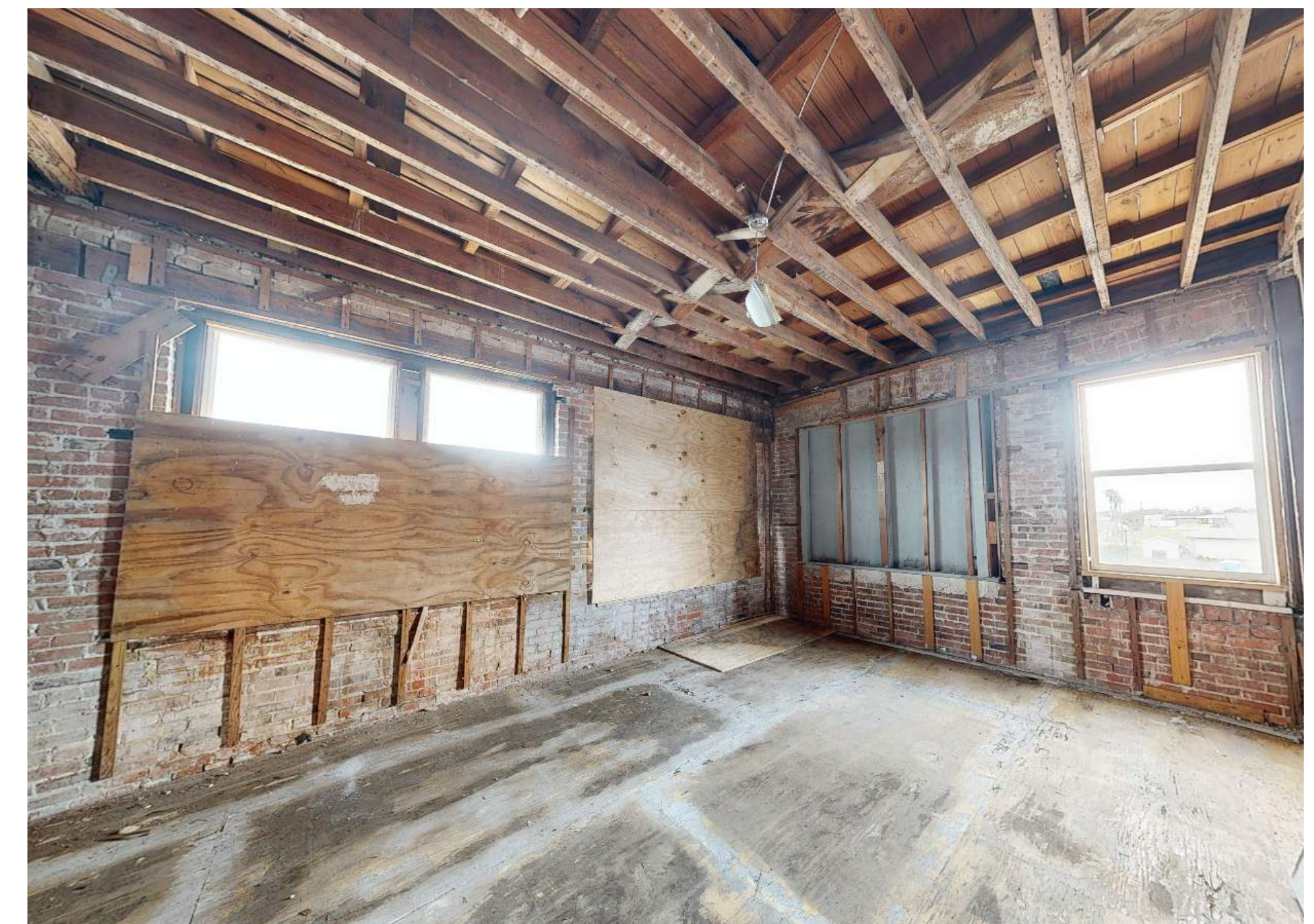
EXISTING INTERIOR - BAY 4 - LEVEL 2
