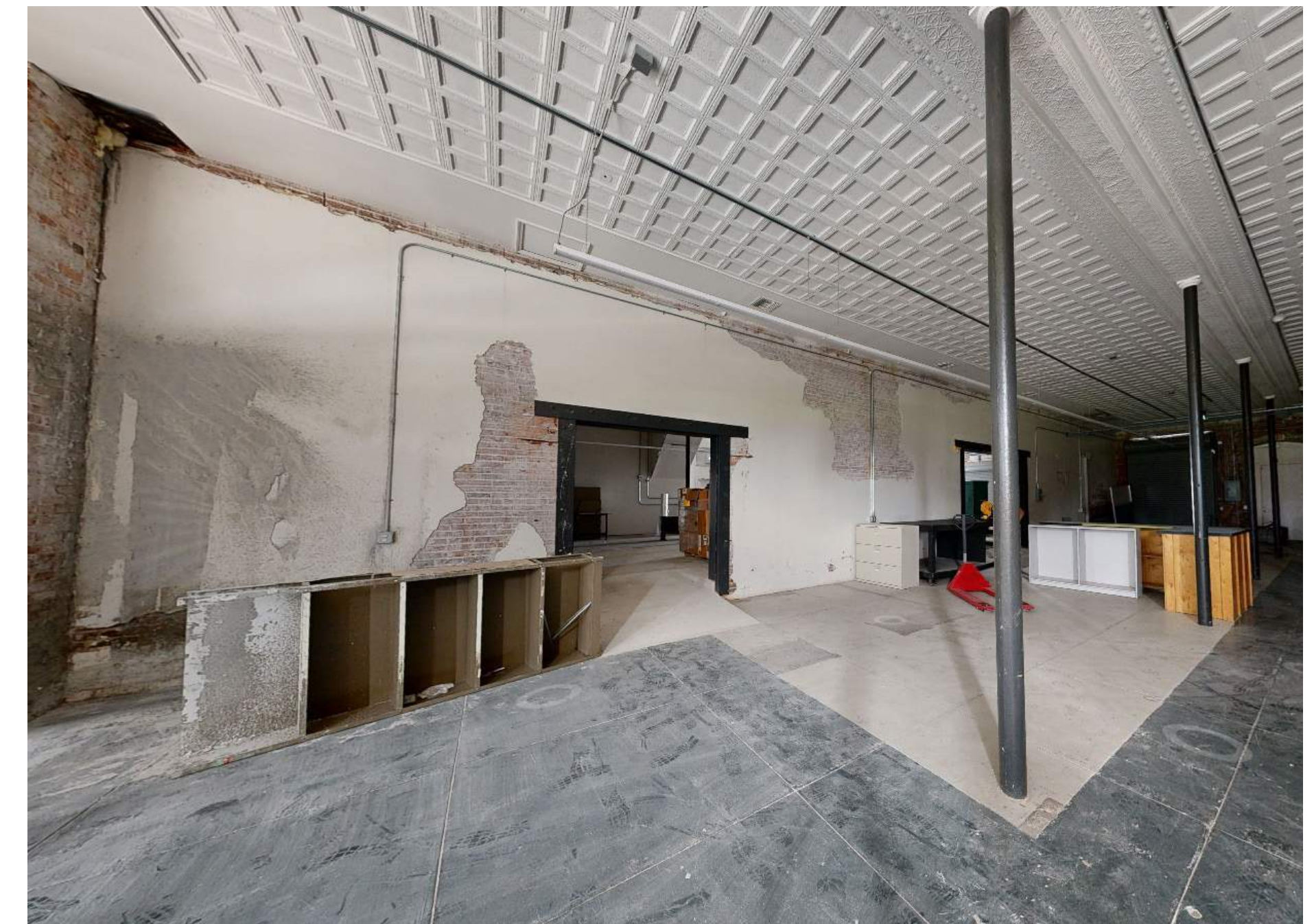
EXISTING INTERIOR - BAY 3
