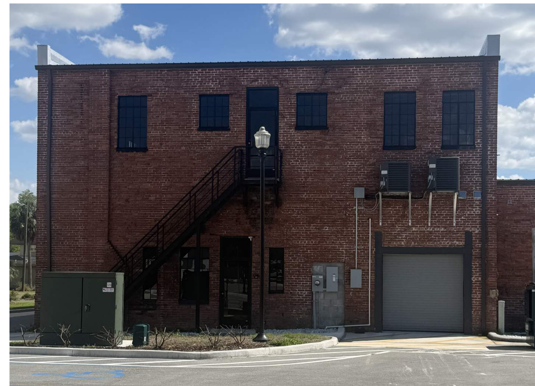
EXISTING SITE - NORTH BUILDING FACADE (BAY 1)
