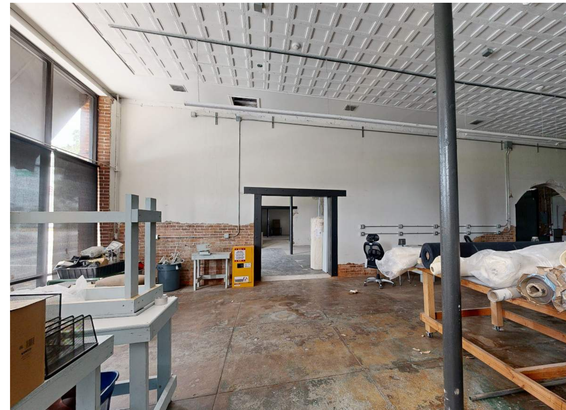
EXISTING INTERIOR - BAY 2
