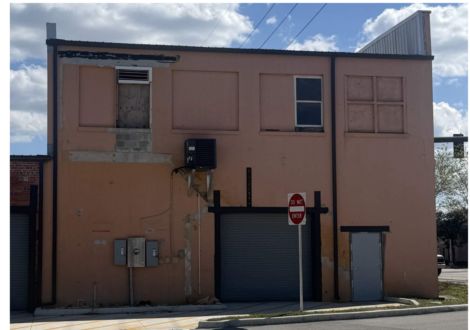
EXISTING EXTERIOR - NORTH BUILDING FACADE (BAY 4)
