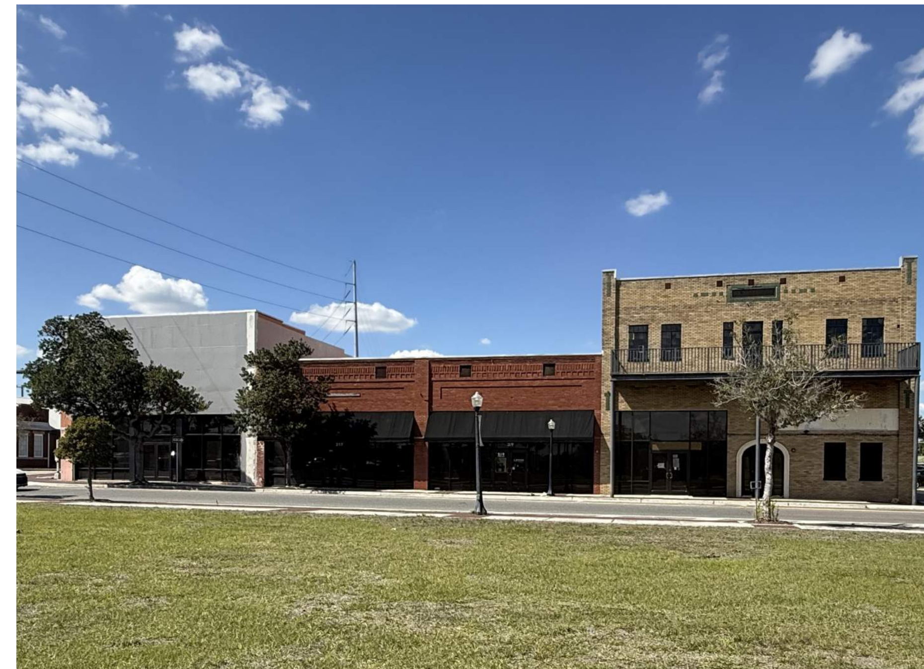
EXISTING EXTERIOR - E MAIN STREET
