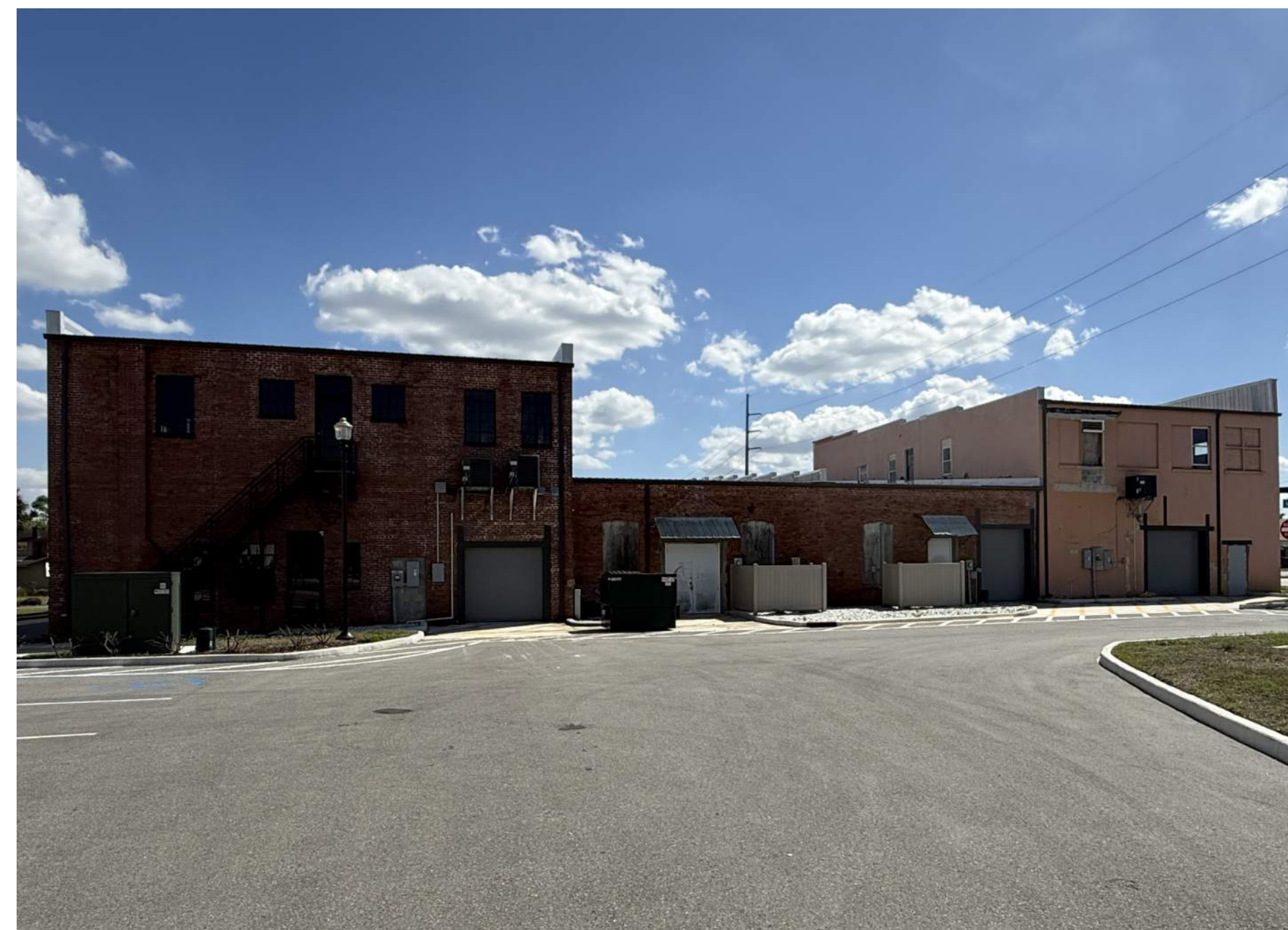
EXISTING EXTERIOR - NORTH BUILDING FACADE
