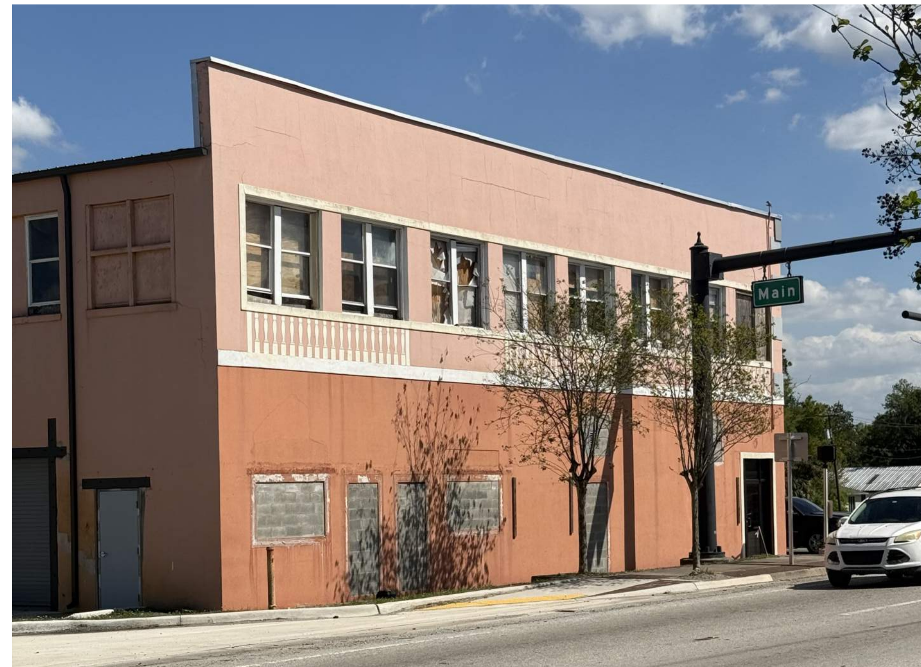
EXISTING EXTERIOR - US 17 N (BAY 4)
