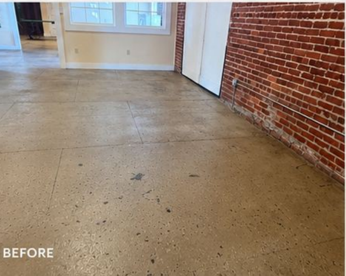
AFTER MOCK-UP CEMENTITIOUS OVERLAY WITH MATTE SEALER
