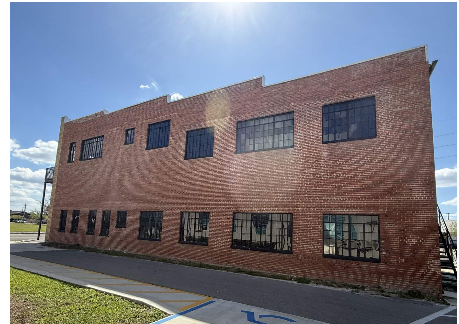
EXISTING EXTERIOR - EAST BUILDING FACADE (BAY 1)
