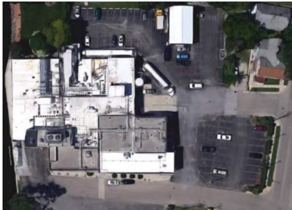
Figure 5: Aerial of Existing Plant
