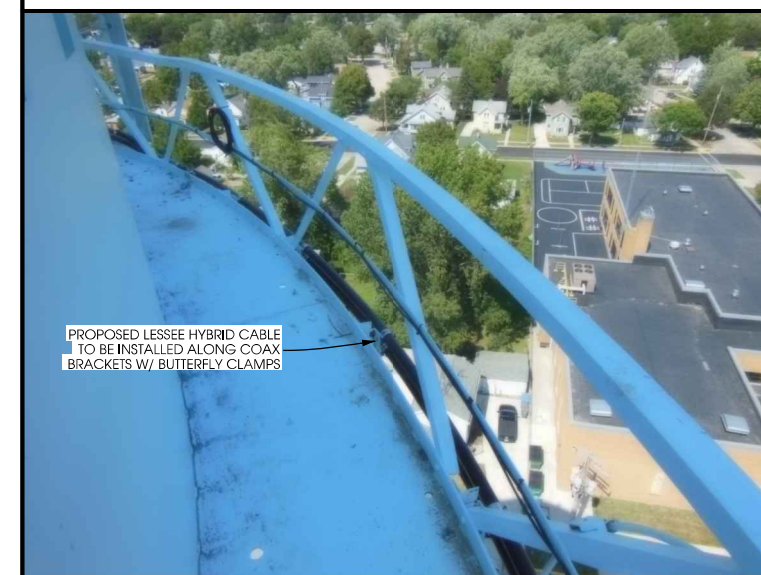
EXISTING CATWALK RAILING
