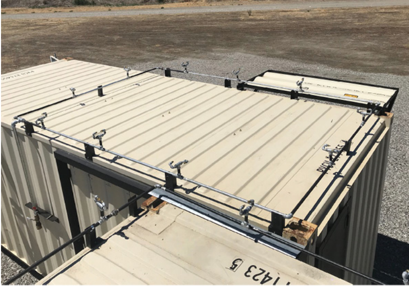
(12) Exterior sprinklers protect the container and reduce interior temperatures between evolutions. (Photo courtesy of 3sFire.)
