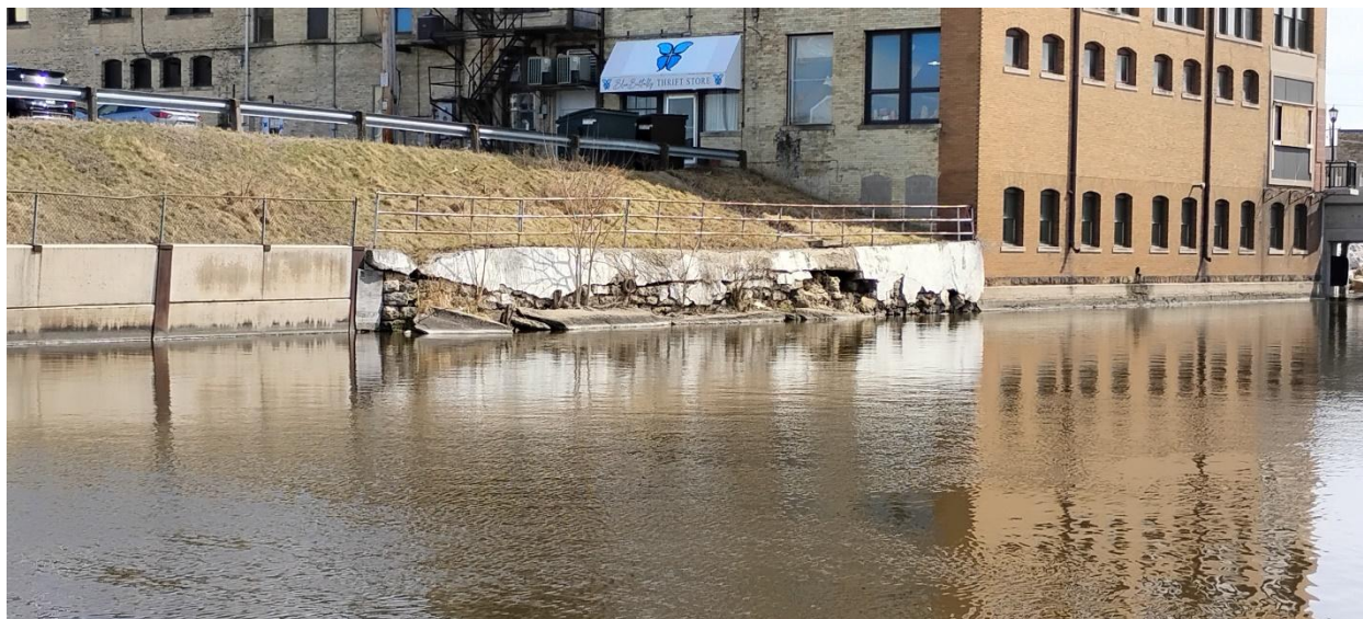
Figure 2. View of Section A looking southeast.
