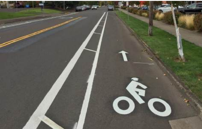
Bike Lane Example with buffered stripe markings
