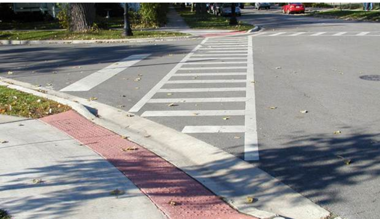
Curb ramp with crosswalk markings
