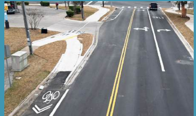
Curb ramp from on-street bike lane
