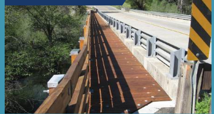
Bike and pedestrian bridge addition
