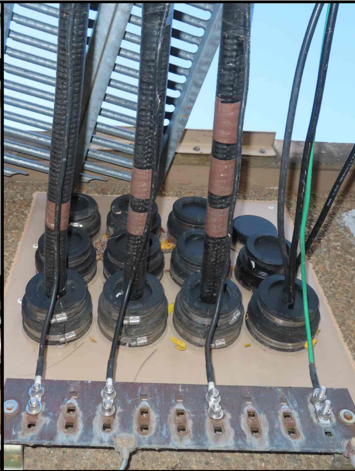
D SHELTER COAX PORT (SHELTER EXTERIOR)
