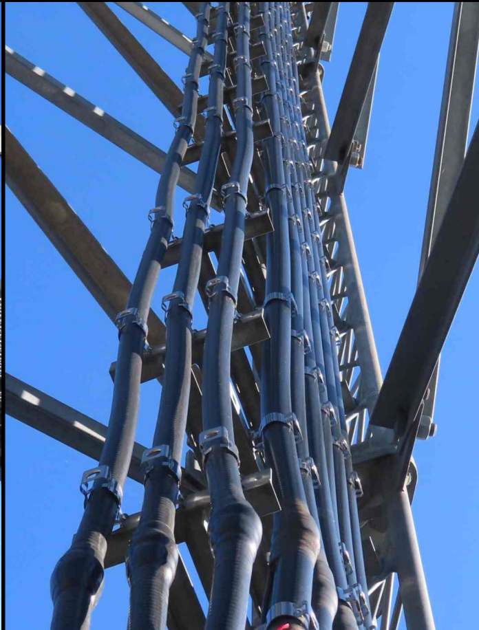
F CABLE ROUTING UP TOWER LEG B
