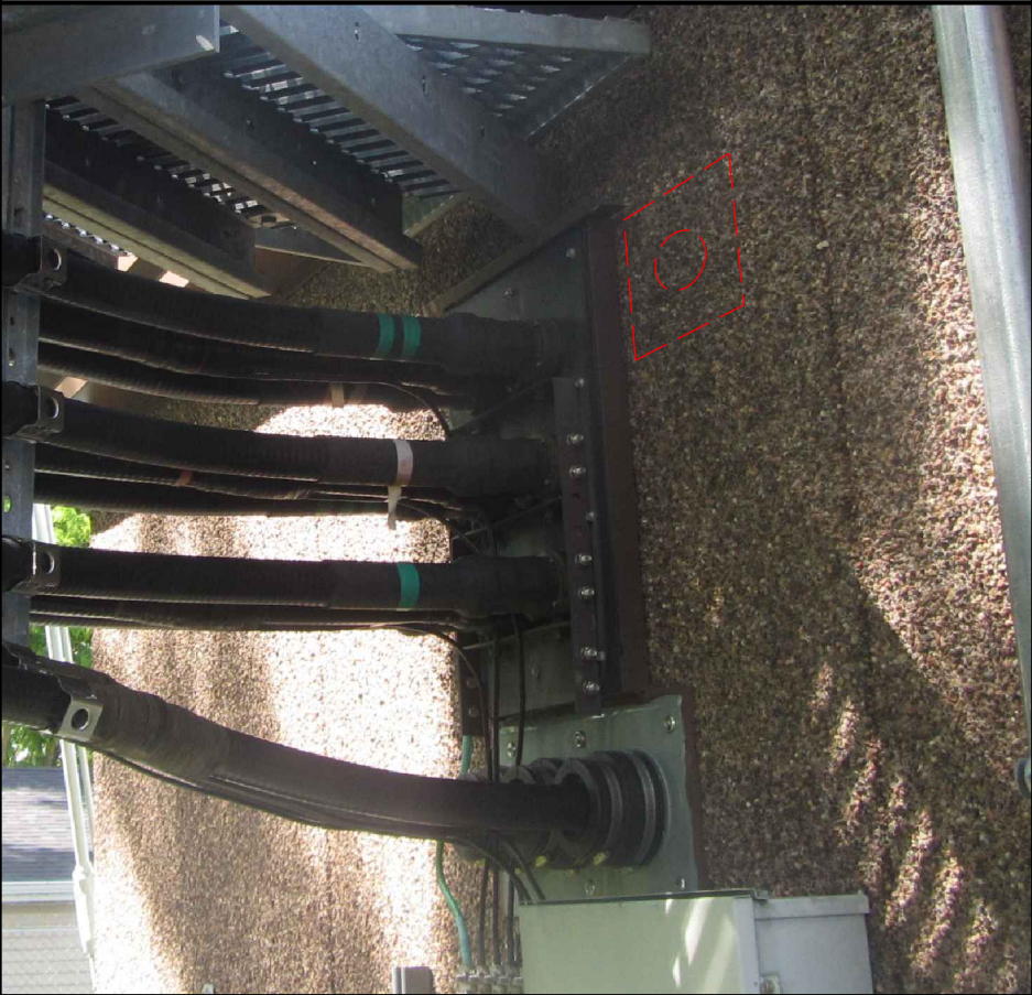
EXISTING COAX ENTRY PORT - EXTERIOR
