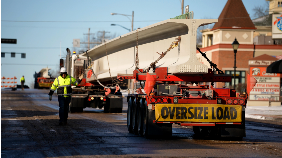
Girders being delivered for the Main Street (Cole) bridge project, January 2025.
