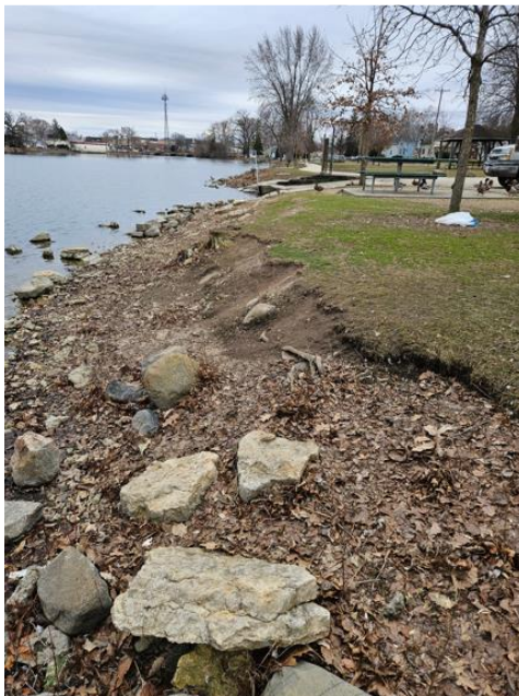
Photo 2 (facing south along shoreline) near parking lot.
