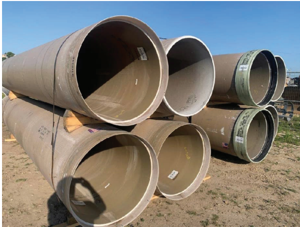
Thirty-six-inch Hobas FRP Sanitary Sewer.
