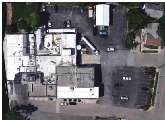
Figure 5: Aerial of Existing Plant
