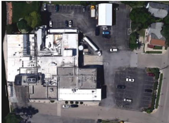
Figure 5: Aerial of Past Plant
