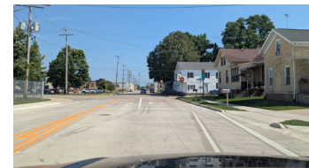
Existing bike lane
