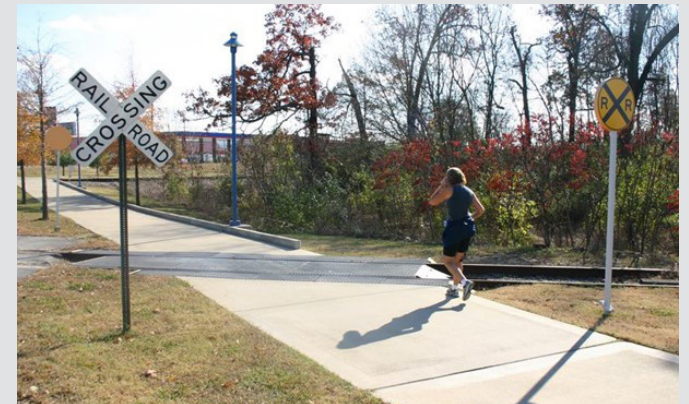
Signage and trail surface shown, along with an angled crossing in Chattanooga, Tennessee
