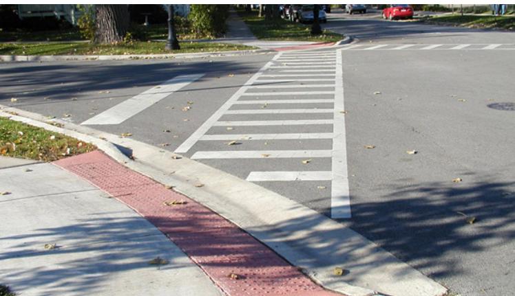
Curb ramp with crosswalk markings
