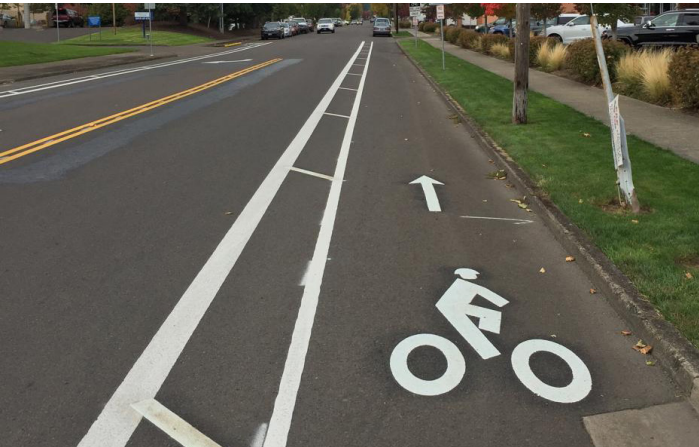
Bike Lane Example with buffered stripe markings
