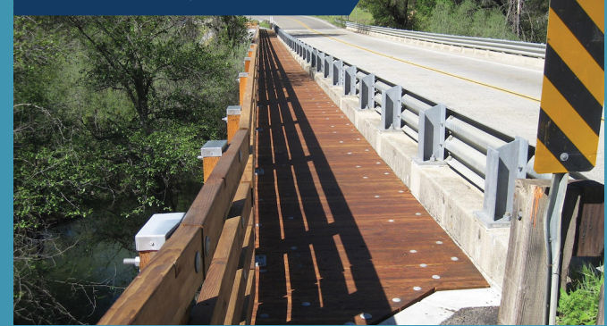
Bicycle and pedestrian bridge addition to a roadway bridge
