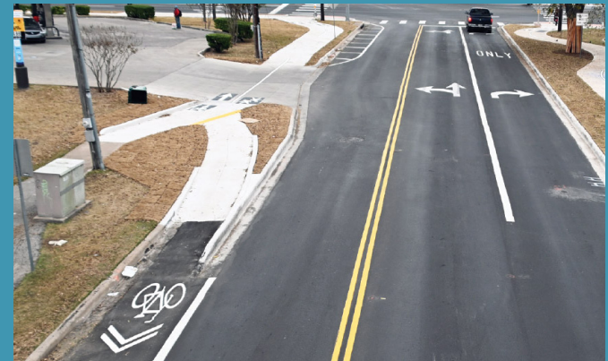
Curb ramp from on-street bike lane
