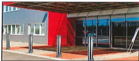
Internal Locking Bollards – A cam lock near the top of the bollard secures the locking mechanism into the embedment sleeve.
