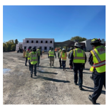
WFD Staff toured the progress of the new station
