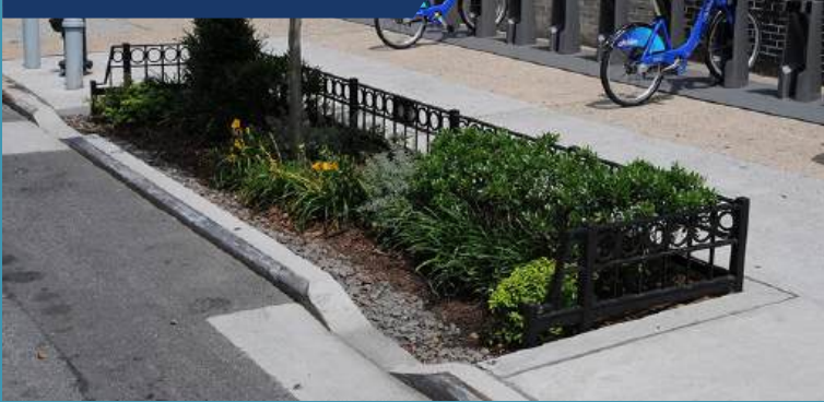
Rainwater garden and curb cuts
