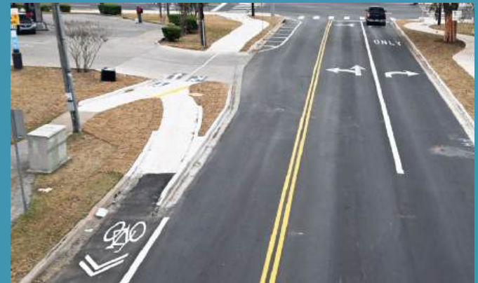
Curb ramp from on-street bike lane
