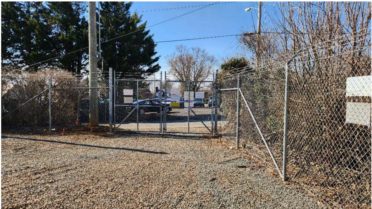
Picture 2 - Example photo of existing security fence.
