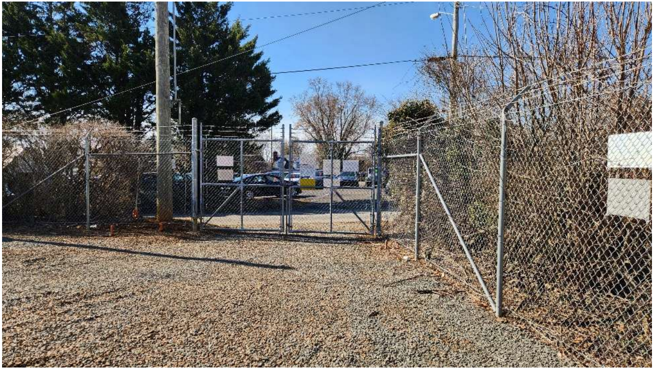
Example photo of existing security fence
