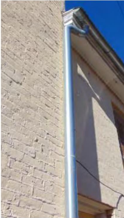
Figure 3-43: This galvanized steel downspout is not historically appropriate. To comply with the guidelines, the downspout should be painted to blend in with building.
