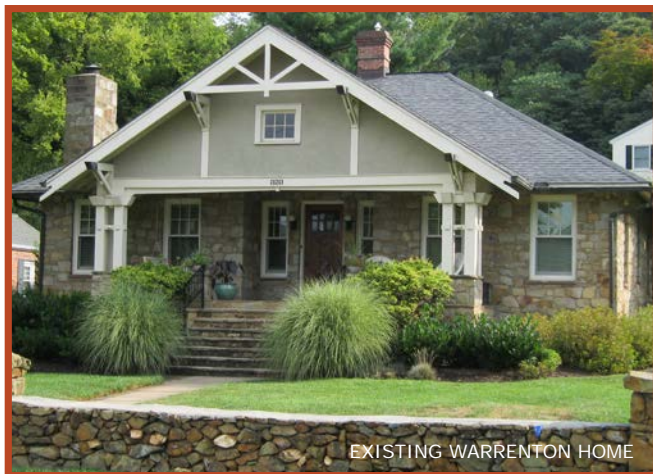
Exposed Rafter Tails and Knee Braces
