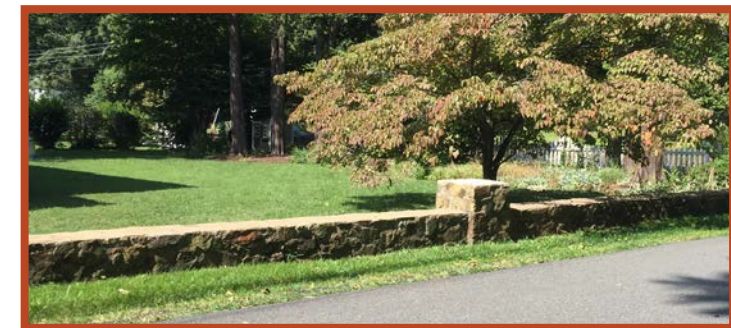
STONE COLUMN & WALL
