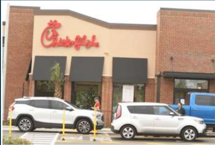
Customers go through the new drive through lanes at the Chick-fil-A store in Hanover Center Friday Nov. 6, 2020 after renovations were completed this week. The inside of the Chick-fil-A remains closed to diners due to concerns over COVID-19. (KEN BLEVINS/STARNEWS) WIS
