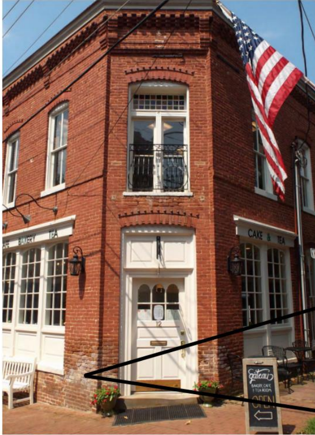
Figure 3-23 Salt efflorescence is a sign of nemetual moisture on masonry surfaces
