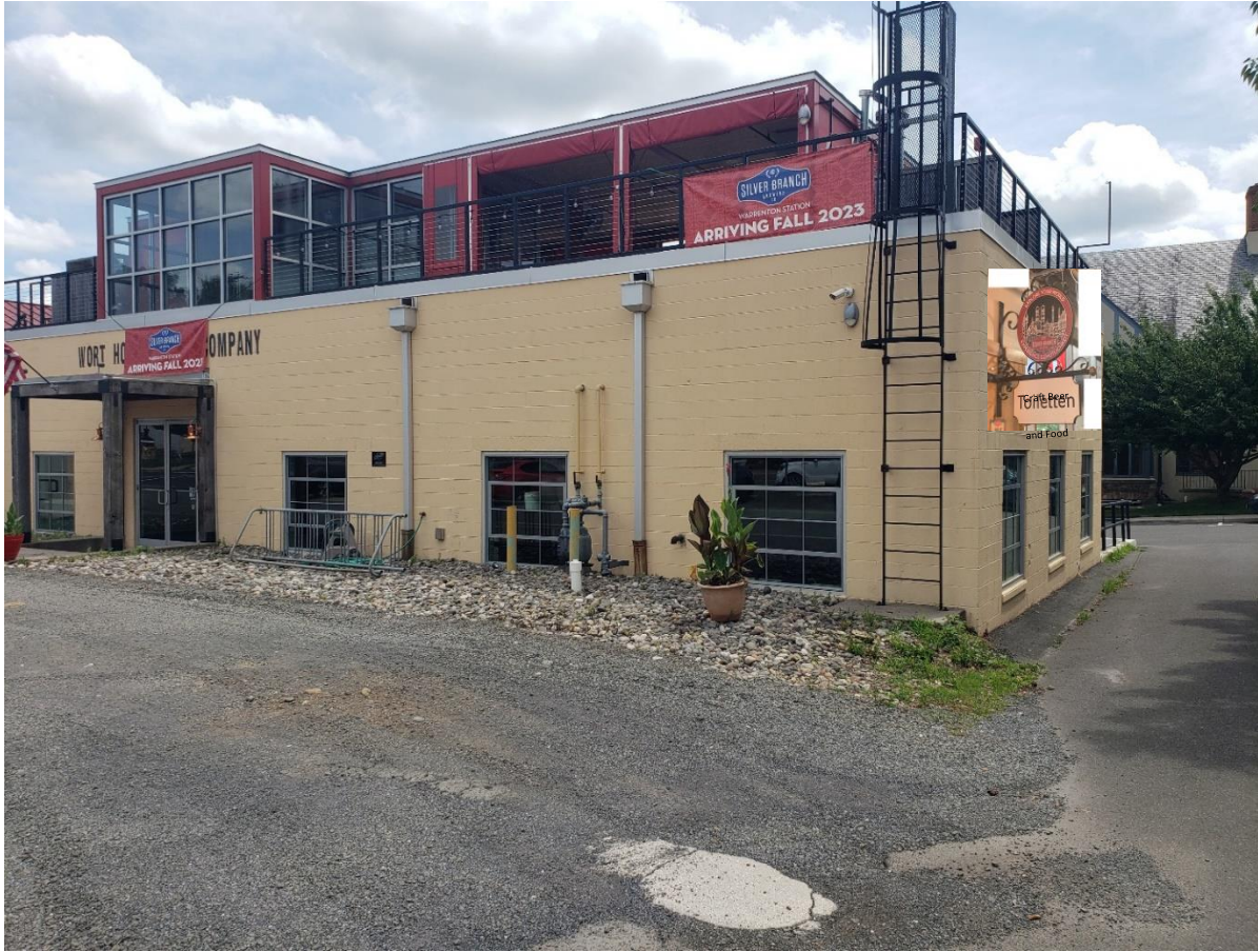
Projecting sign on the corner of 2 nd Street
