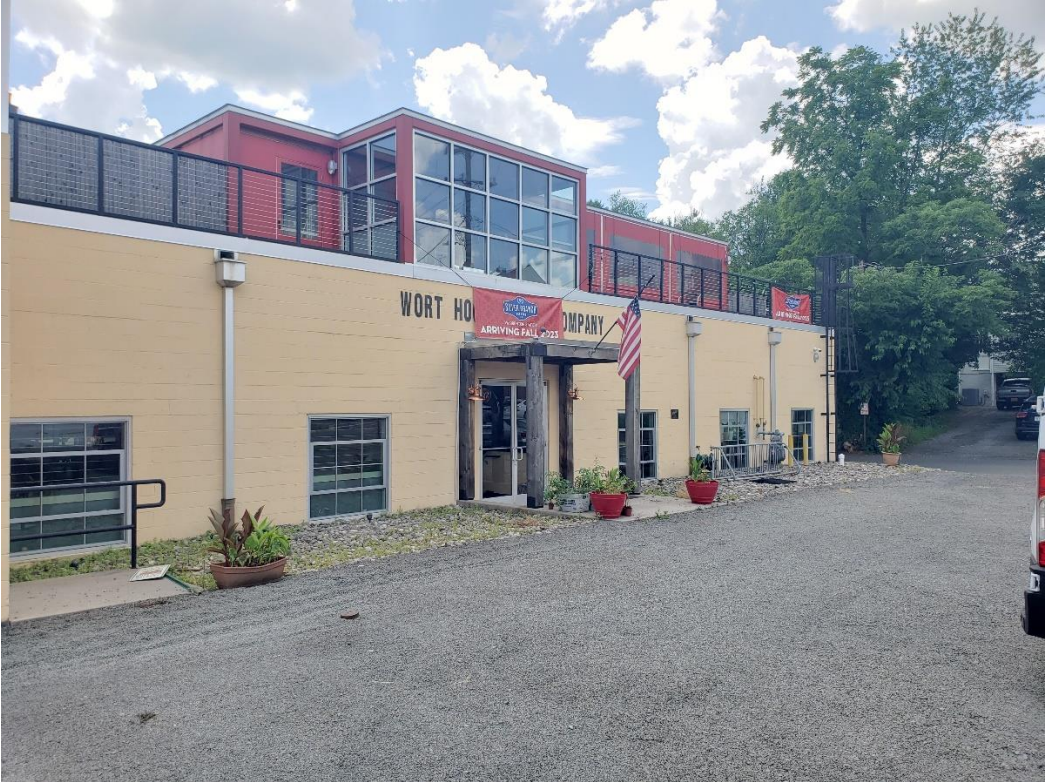
1) Replace painted sign on Lee Street side of 41 Beckham Street.
